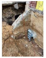
in helping address the large footings, but not a complete solution. The team also relied on cutting the concrete and shoring the foundation with temporary support props. By utilizing all these tactics together, they were able to successfully restore the high school to its former glory.
