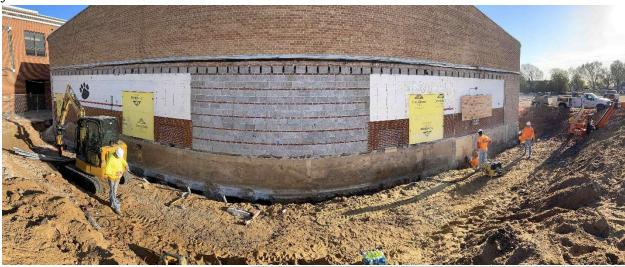
The crews faced multiple challenges during the two-week project. One such obstacle was the large footings, and properly benching the soil. To safely protect the team from cave ins, they excavated the sides of the trenches with a series of horizontal levels using a method called benching. Safety protocol dictates
