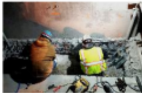
Technicians are preparing the transformer footing for bracket installation.
