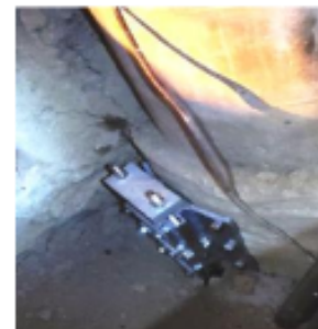
This is a view of a completed pier installation on a caisson.
