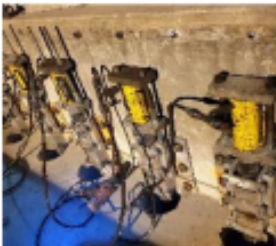
Hydraulic jacks are used to lift the transformer and footing.
