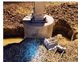
The special concave column mounted bracket is shown.
