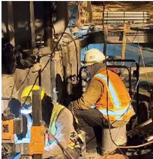
Workers are installing wall mount pier brackets on the transformer footing.
