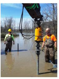
There were a total of 902 vertical *ECP Torque Anchor*™ compression piles and 228 helical anchors installed for lateral support on the project. The large number of placements and short time frame dictated
