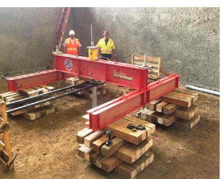
There were two tension load tests performed, one in each basement. The tests were performed to ASTM D1143 standards along with procedures recommended by ECP. The entire testing process was supervised by a JPC Engineering inspector.
