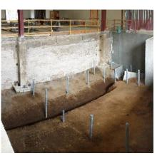
The helical pile installation was accomplished using a Pro-Dig X20K hydraulic torque motor attached to a mini-excavator. Shaft torsion was used to estimate pile capacity during installation and later pile capacity was verified by load testing.
