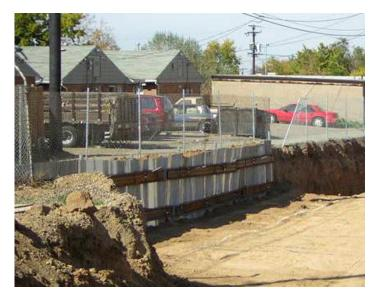
A new multi-housing unit was planned on this site. The plans called for the new foundation excavation adjacent to a public street. The engineer called for temporary shoring to stabilize the soil cut, and to support the road during This project required installation of two different helical screw pile products. The Torque Anchor installations and shoring construction had to accomplished in stages to prevent loss of soil support from beneath the road.
