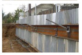
construction progressed, two rows of Model TAF-150 ECP Square Bar Tiebacks were installed with center to center spacing of ten feet. This spacing coincided with the tubular piles. Horizontal support for the steel decking was accomplished by installing C12x30 steel channel beams as a waler system for the two rows of tieback anchors.
