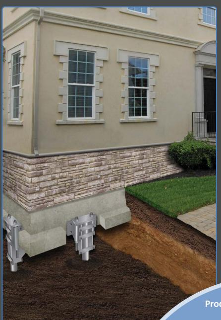
The ECP Steel Push Pier System is a permanent solution for your home's settling foundation. It provides you the very best option to repair your foundation back to level. Steel piers are hydraulically driven through our patented steel bracket to a load bearing stratum, as the entire structure works as the reaction.
