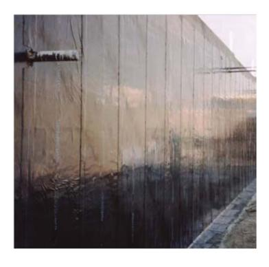
CCW MiraDRI self-adhering membranes are composite materials consisting of a specially formulated rubberized asphalt laminated to a high-impact resistant HDPE film. The CCW MiraDRI waterproofing system is designed to provide waterproofing protection for below-grade foundation walls, slabs, parking decks, plaza decks, tunnels and many applications. The CCW MiraDRI waterproofing system consists of the self-adhering membrane, and an environmentally friendly water-based primer for surface preparation
