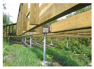
Timber brackets, fabricated from stainless steel, were used to attach the pile shafts to the bridge girder beams. Set screws on the bracket sleeves provided uplift restraint on the foundation piles.
