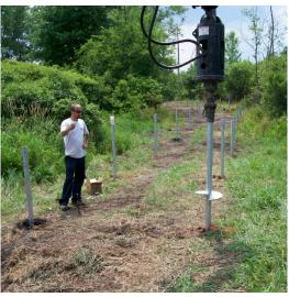
The lead section consisted of a seven foot long shaft that had a 12 inch and a 14 inch helical plate attached on the bottom. The lead section was followed by seven foot or ten foot extensions to achieve the installation depth requirement plus sufficient shaft height for attachment the bridge structure. The specifications required that all shaft connections occur below grade.
