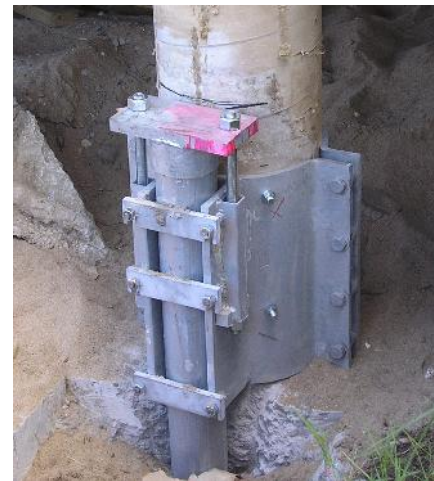
This is a view of the Model 450-WM (12" Dia.) bracket that connects the 4-1/2 inch tubular pile shaft to the 12 inch diameter concrete column.
