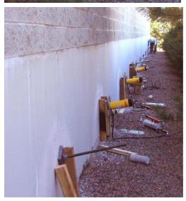
Helical Torque Anchors<sup>™</sup> were installed to provide supplemental lateral wall support and to restore the stem walls plumb (vertically upright). All of this work had to be accomplished while the retail business remained open.
