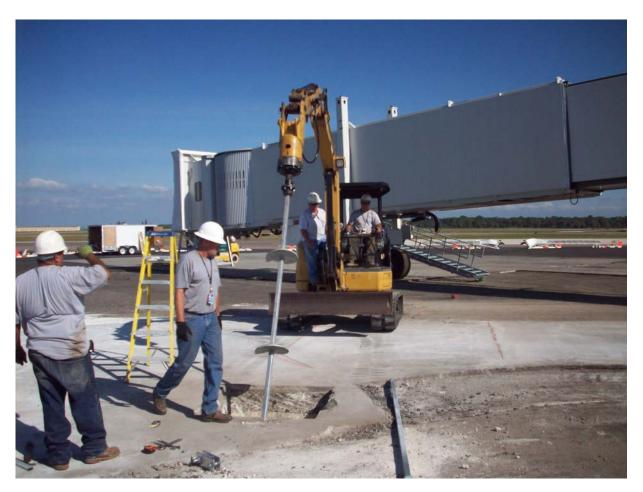
The photograph above and on the previous page shows the installation of the ECP Torque Anchors  $^{\text{\tiny TM}}$  at one of the new passenger bridges. The tieback anchor configuration consisted of three 14 inch helical plates attached to a 1-3/4 inch high strength square shaft. The anchors were advanced into the soil using a 12,000 foot-pound hydraulic gear motor shown mounted to a mini-excavator's dipper arm.
