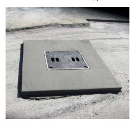
The entire project took only two days to complete. Once the tiebacks were installed and accepted, the attachment couplings were installed. Finally, the access frames were cast into a new concrete pad and the covers installed to complete the project. N Square's proposal to use helical screw piles resulted in a substantial savings to the customer, and delivered the finished product in about one-third the time of the alternate design.
